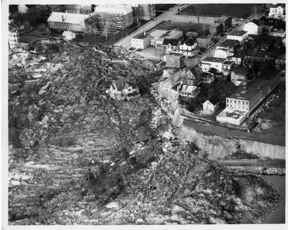
Figure 6 : Homes destroyed or partially destroyed. Like in figure 1, note on the right side of the photo the path leading to the toe of the riverbank, with a very steep slope. (Source : Canada Wide Photos)
