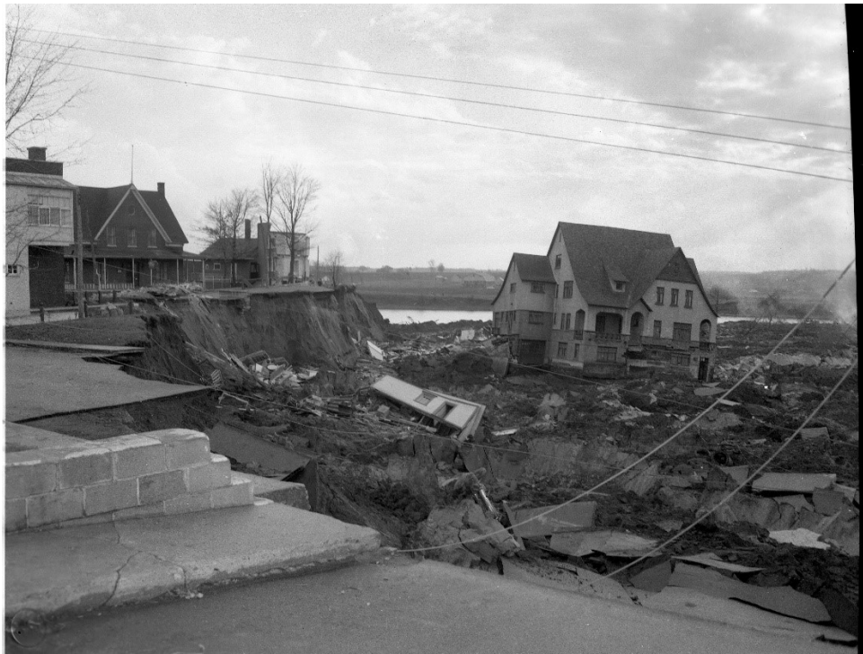
Figure 5 : Home built on a foundation raft that remained intact in the scar left by the landslide. (Source : Appartenance Mauricie, 3042-074)
