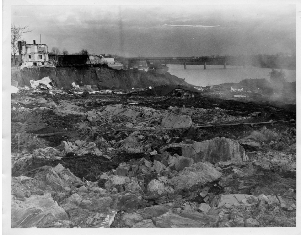
Figure 19 : Debris partially remolded in the scar. Two horsts are visible on the right side of the photo. (Source : Ministère des Transports et de la Mobilité durable, H. A. Beaudouin)
