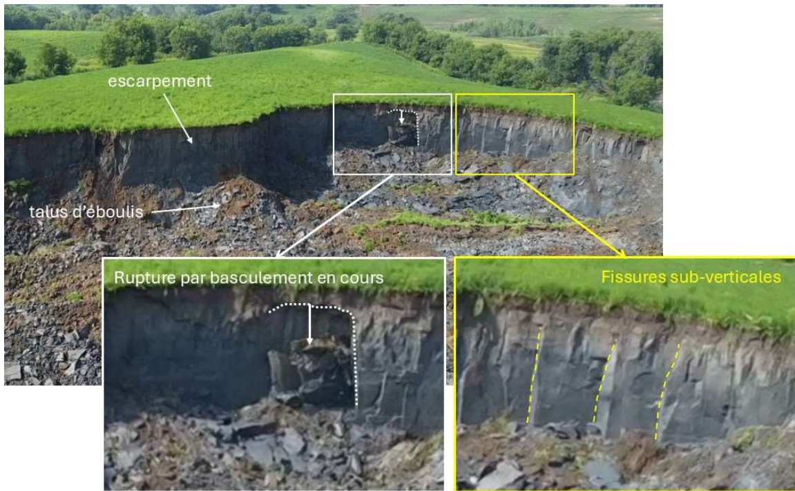
Figure 9: Drone photos from July 16, 2025, showing subvertical cracks around the scar, facilitating toppling failures. (Source: MTMD)
