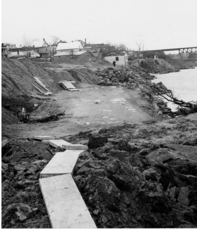
Figure 16 : Work in progress: riprap at the foot of the slope and cut in the slope. (Source : Ministère des Transports et de la Mobilité durable)
