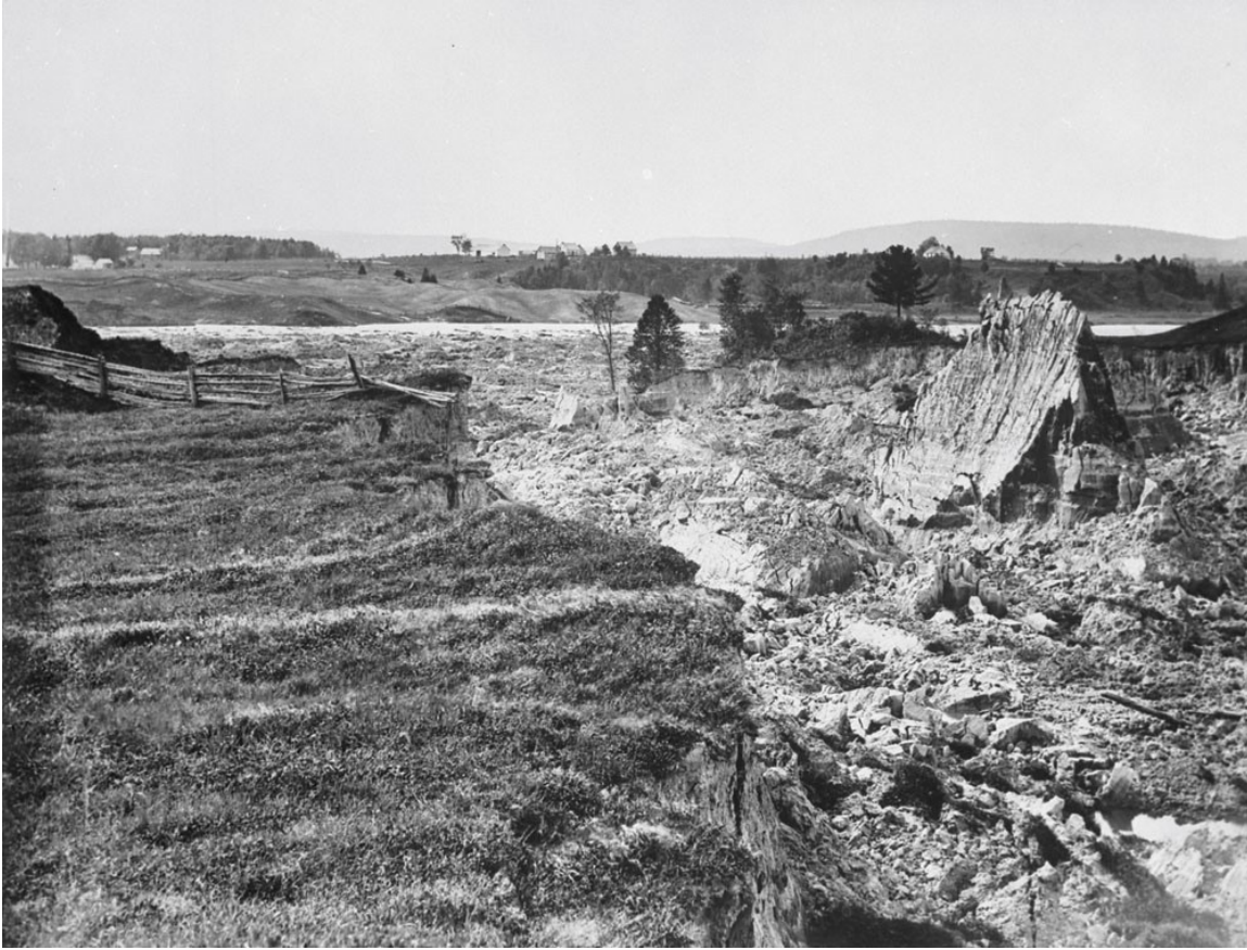
Figure 4: Historical photograph showing a horst in the 1898 landslide. View facing the bottleneck part of the slide. (Source: Library and Archives Canada, PA-050914)
