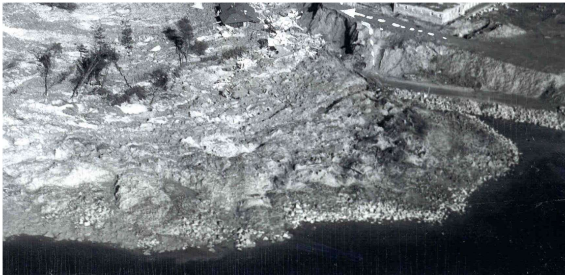
Figure 18 : Riprap swept away by the flowslide and cut in the slope. (Source : Gouvernement du Québec)
