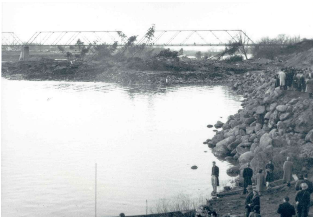
Figure 17 : Riprap upstream from the landslide and debris from the landslide. (Source : Ministère des Transports et de la Mobilité durable)
