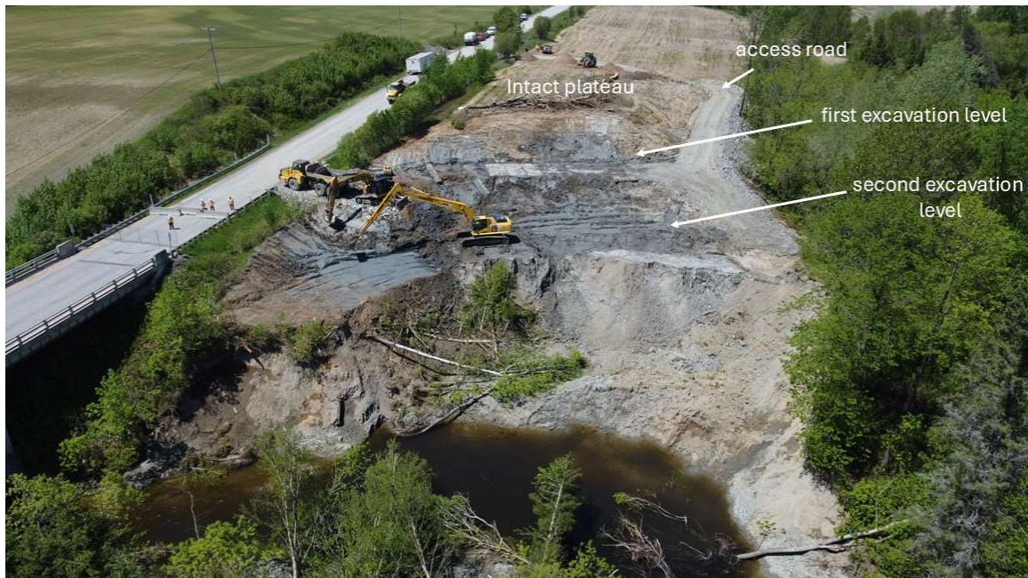
Figure 7 : Excavation of ground levels gradually approaching the landslide scar. The access road was placed in a location where it was lower than the adjacent intact plateau. (Source: MTMD – DGG)
