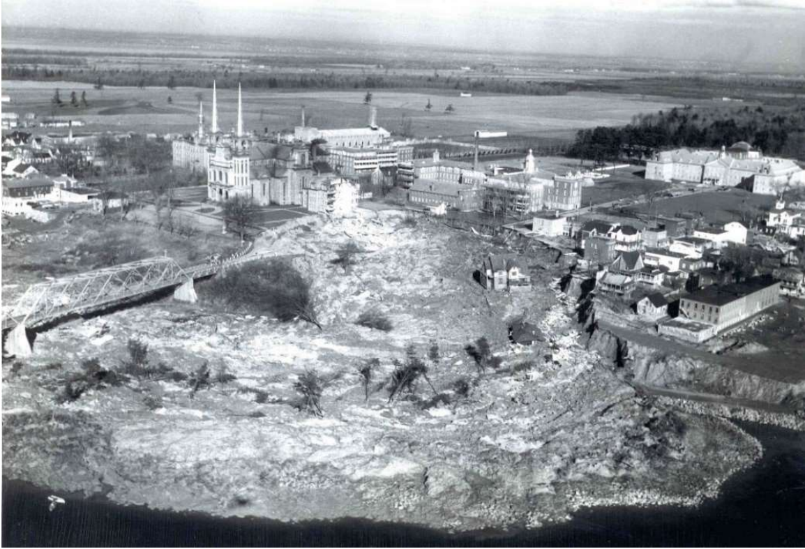
Figure 1 : Overview of the 1955 landslide. Note on the right side of the photo the path leading to the toe of the riverbank, with a very steep slope. The riprap previously laid at the base of the riverbank is visible at the end of the debris on the right side of the photo. (Source : Gouvernement du Québec)
