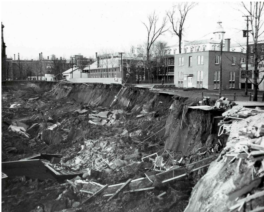
Figure 3 : Backscarp northeast of the scar. (Source : Canada Wide Photos)
