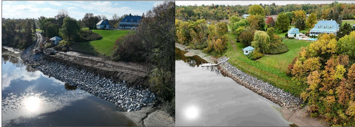
Figure 13 : Stabilization work opposite Rue des Brumes, on the Batiscan River. Left: work in progress. Right: 11 months after completion of the work.
